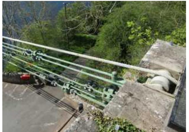
View from the top of the English tower showing the wire rope entering the anchor block over roller bearings.
